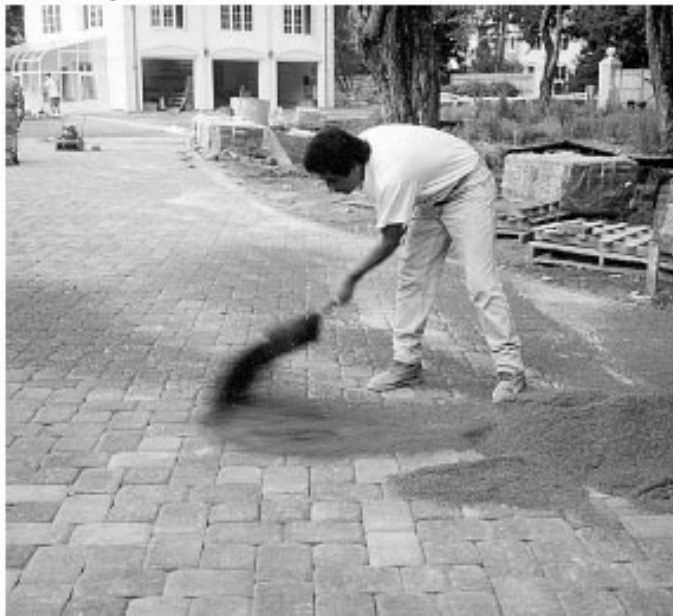
Figure 8. Spreading joint sand over the installed concrete pavers.
